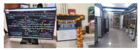
2.0 **Jetha chandan**, **Pokran**, **Ashapura Gomat & Marwar Mundwa station** were commissioned with Kyosan make **Electronic Interlocking** with centralized architecture in Phalodi- Jaisalmer section of Jodhpur division by replacing Std I Semaphore Signalling gears with Std. II(R) by providing the state of the art signaling technology. **With this**
