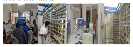
12.0 Conversion of Warm standby EI with Hot standby architecture along with Dual VDU has been commissioned at 20 stations by replacing the existing operating panel of EI system.
