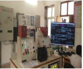
11.0 **Electronic Interlocking** installation with Hot standby arrangement (Kyosan make) and Dual VDU have been commissioned at Zawar stations in connection with Gauge conversion
